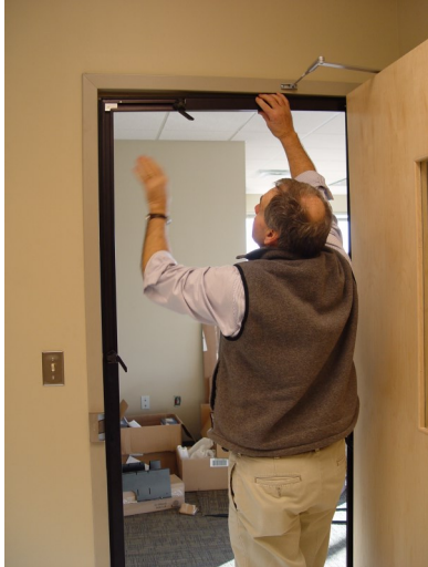
7. Place frame in door for trial fit.
