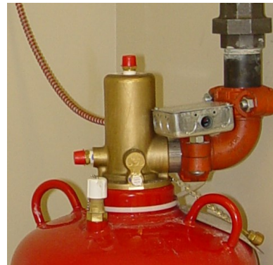
4. First thing—disconnect tank!
