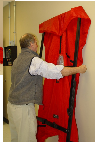
12. Install panel on door frame
