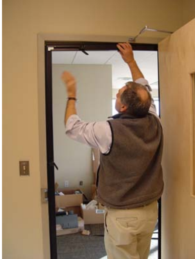
7. Place frame in door for trial fit.
