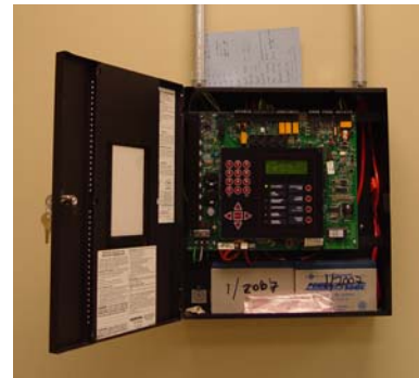
29. Have experience alarm technician, call out alarm system, silence building alarm, and cycle panel to activated any HVAC dampers connected to panel
