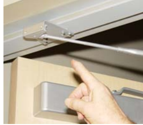
8. If door closer blocks door frame it will have to be removed
