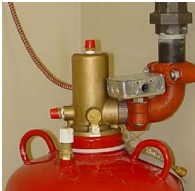
28. Again make sure all tanks are disconnected
